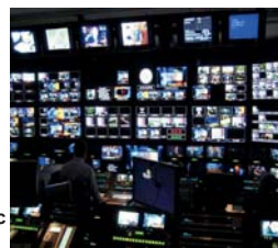
Network Control Room
